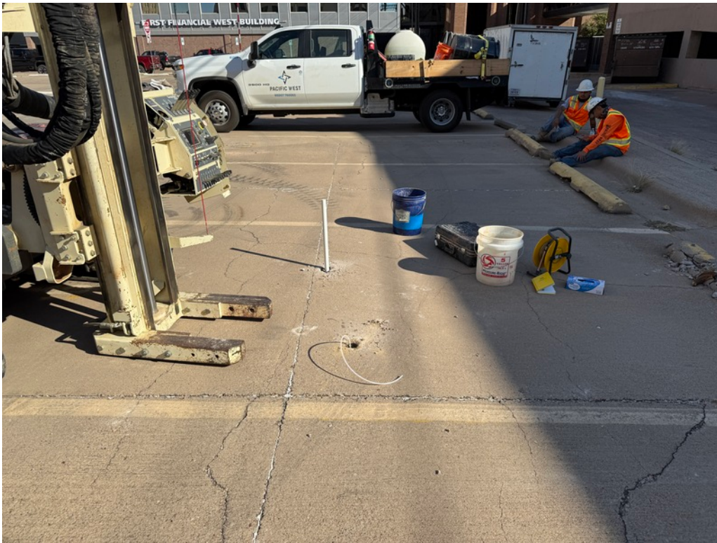
5. (13) View north of TMW-3 and SV-2 soil vapor port
