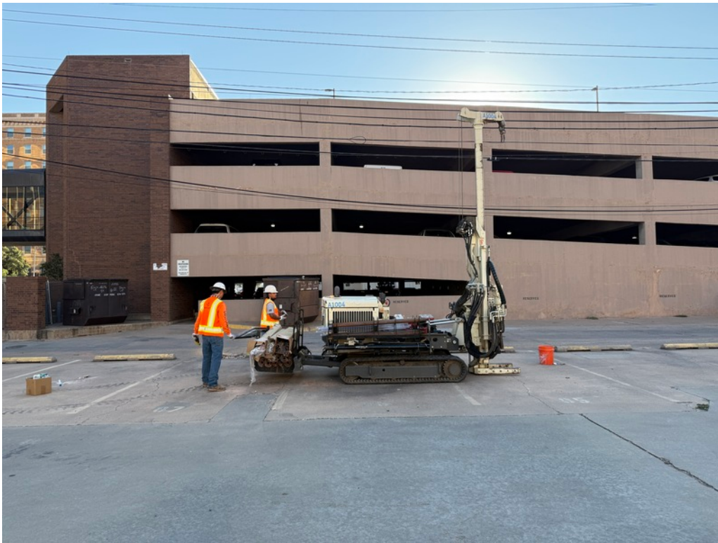
3. (10) View east of SB-2 drilling activities
