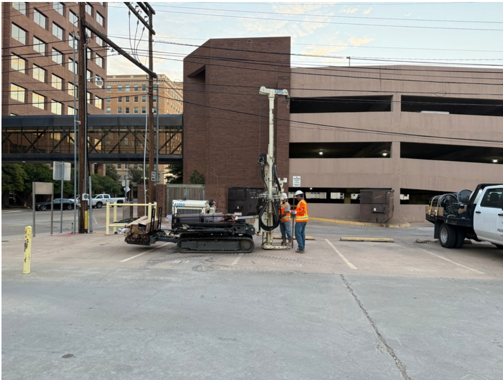
1. (1) View east of SB-1 drilling activities
