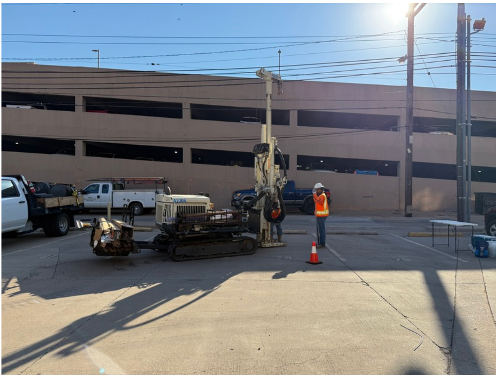
4. (11) View east of SB-3 drilling activities
