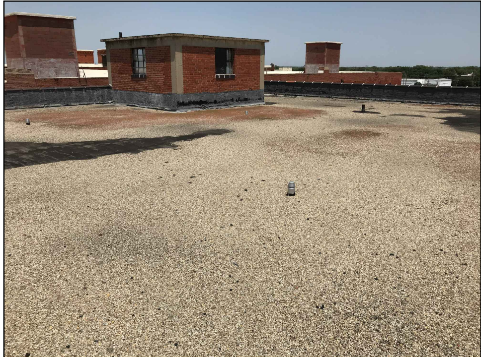
B EXISTING ROOF PHOTOS
