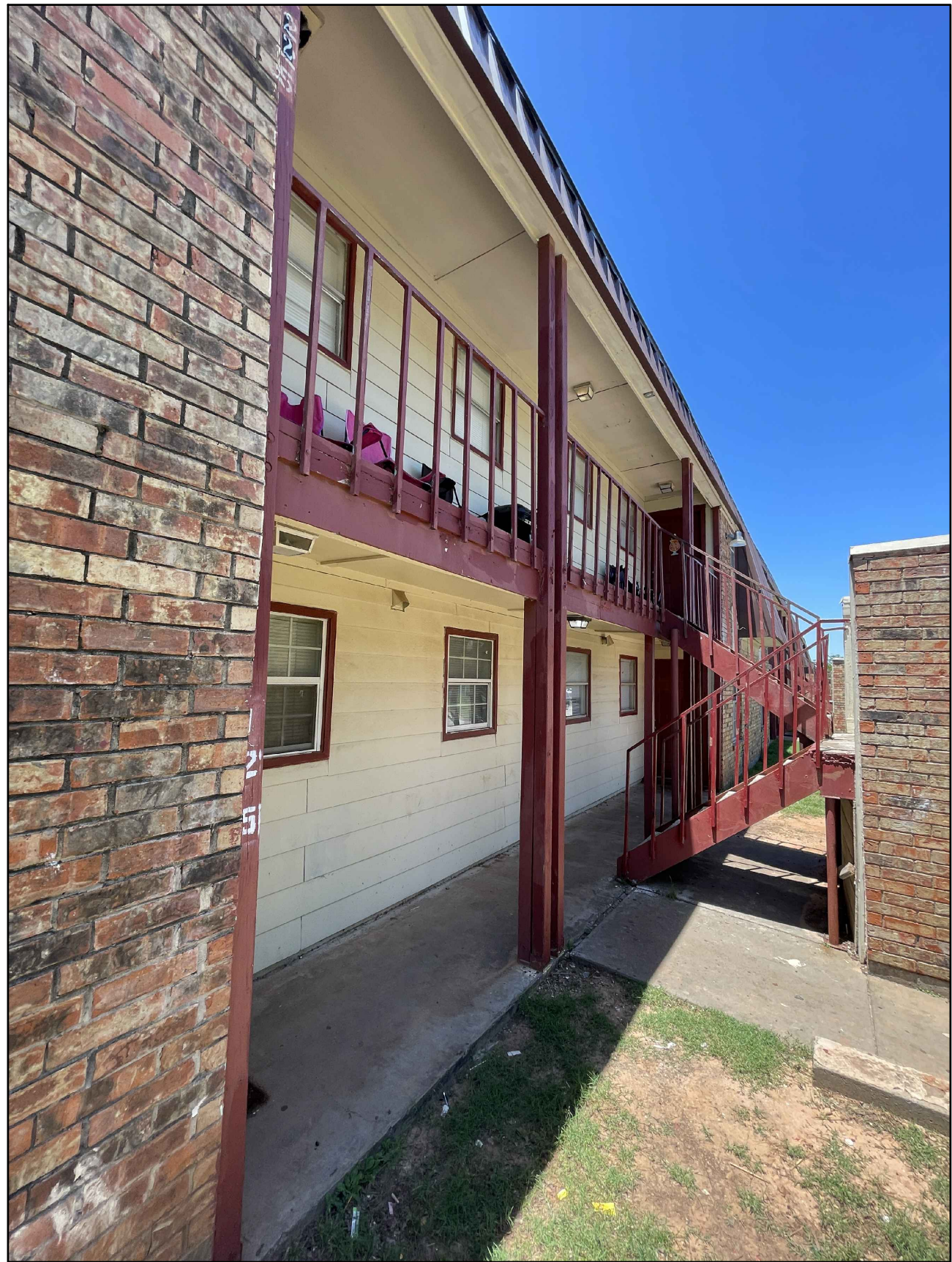
EXISTING CONDITIONS. EXTERIOR STAIR & BALCONY SYSTEMS TO BE REHABILITATED &/OR REPLACED AS NOTED ON A2.13 & STRUCTURAL DRAWINGS. NEW STAIRS, NEW CONCRETE PAD UNDERNEATH STAIR, NEW CONCRETE SLAB AT SPECIFIC BUILDING LOCATIONS NOTED FOR ACCESSIBLE UNIT SLOPES.
