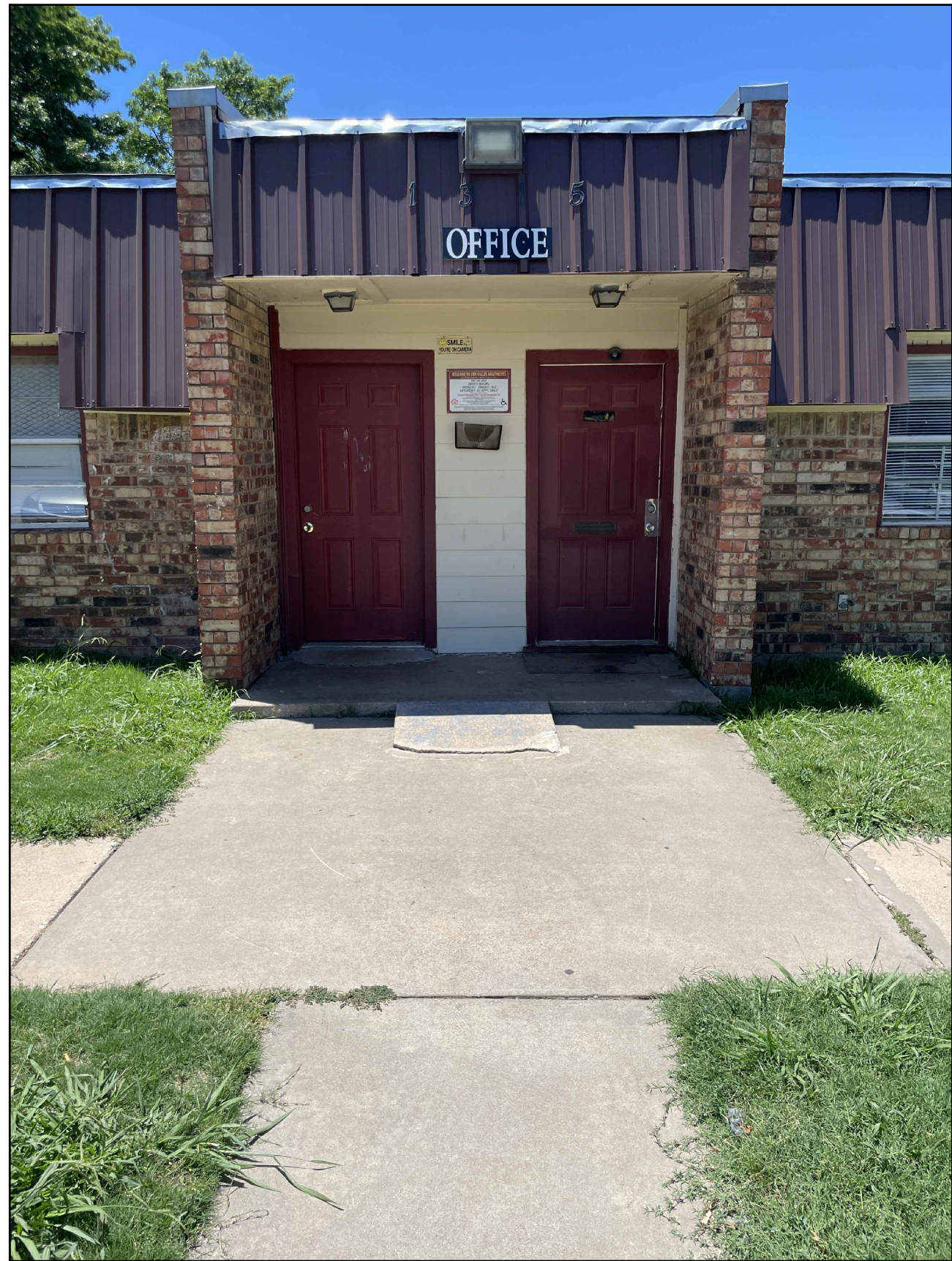
EXISTING CONDITIONS. ENTRY DOORS TO REMAIN. REFERENCE S.O.W. FOR WORK AT CLUBHOUSE EXTERIORS. PER OWNER.
